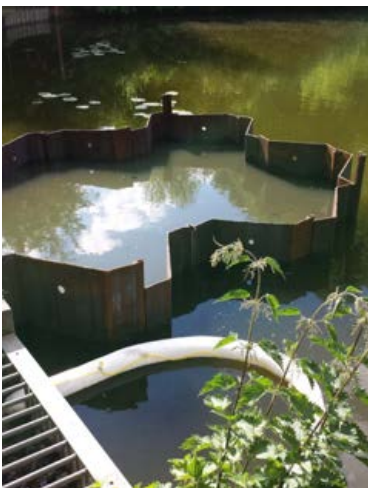
Picture 5 - Temporary coffer dam at Viaduct Pond.
