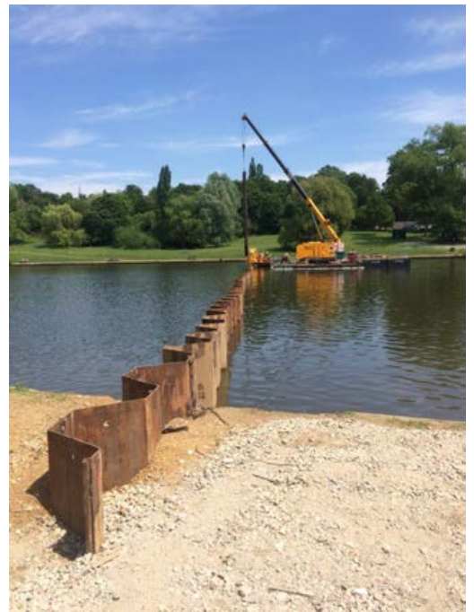
Picture 4 - Temporary dam nears completion at Model Boating Pond.
