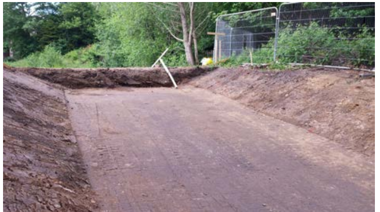
Picture 6 - Spillway under construction at Viaduct Pond.
